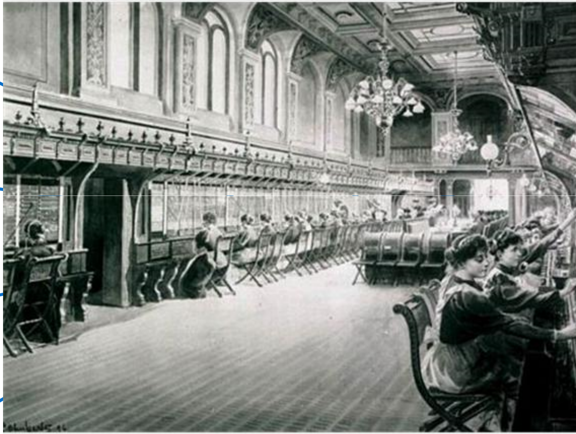
SAT's main telephone exchange, Stockholm 1897 - 7000 lines "Multiple switchboard" - each operator could work independently.
